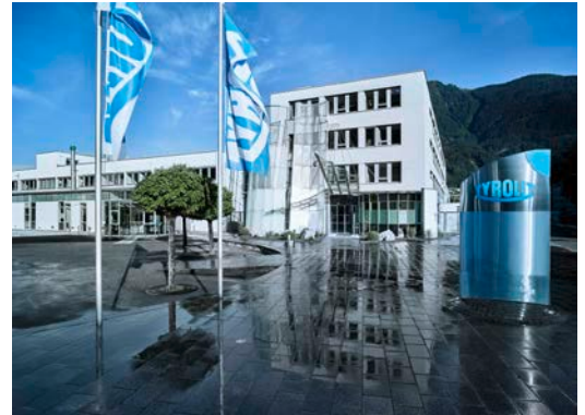
TYROLIT company headquarters in Schwaz, Austria
