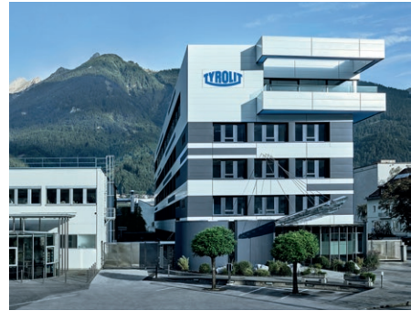
Tyrolit headquarters in Schwaz (Austria)
